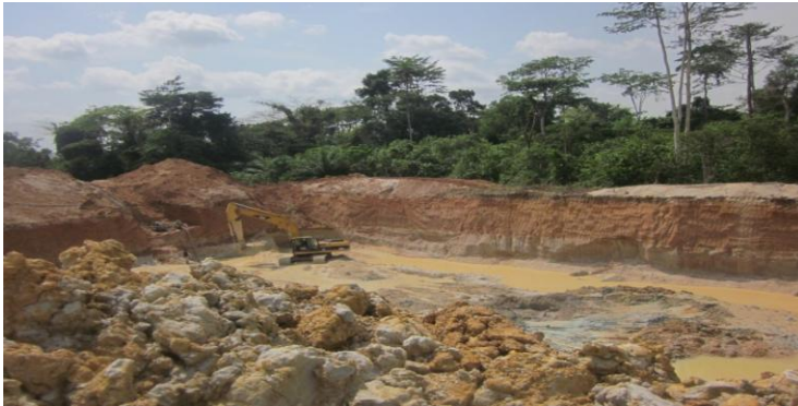
Figure 1. Pit under Construction by an Excavator
