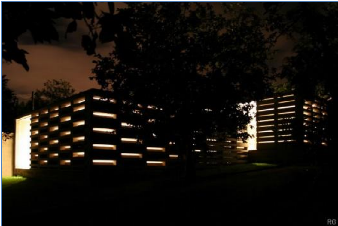
Figure 5: Pentimento House is a great example of the integration of form and function
